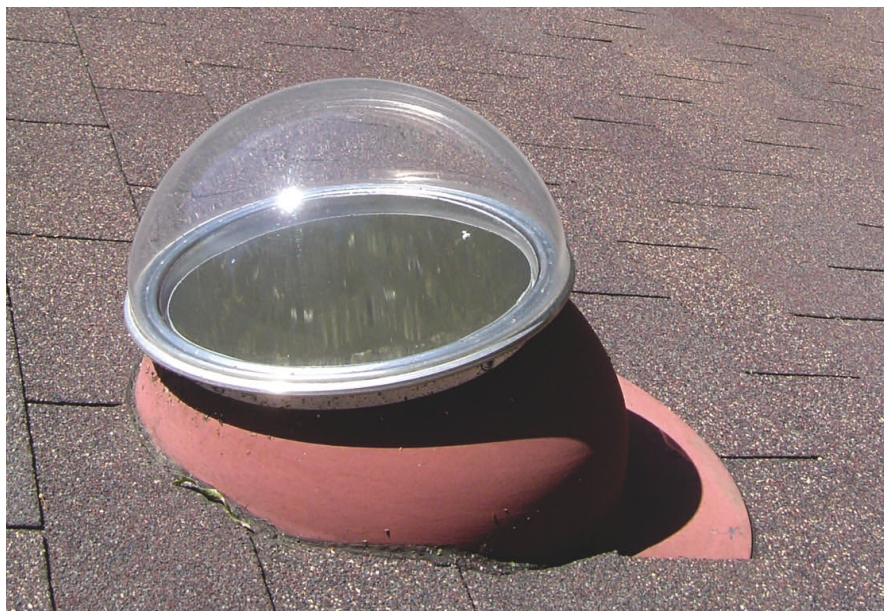
Tubular skylights are generally easier and less costly to install than conventional skylights.
